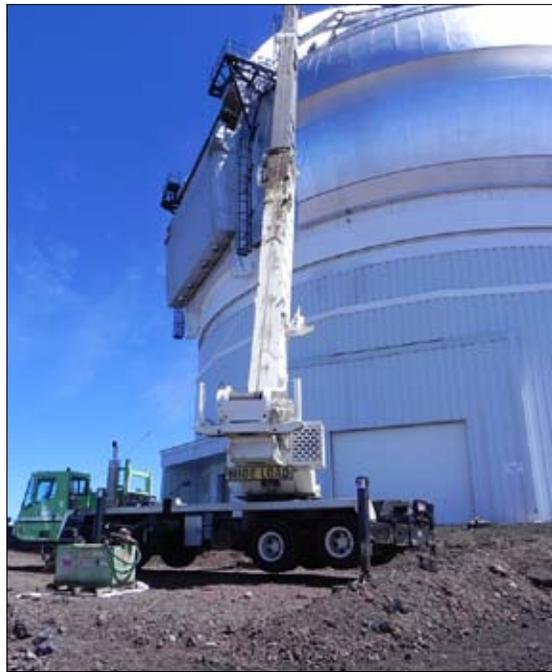
**Figure 3.** A 150-foot telescoping crane was needed to install the Shutter Service Platform.
