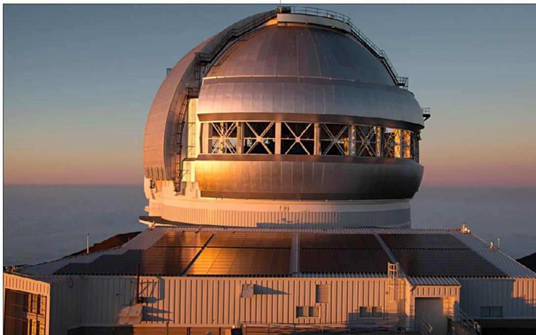
**Figure 2.** Recently installed photovoltaic panels on the Gemini North telescope facility on Maunakea are some of the energy saving initiatives that are part of the Transition Program. Since installation, the panels have provided approximately 10% of the energy needed at the Gemini North telescope. Photo credit: Joy Pollard
