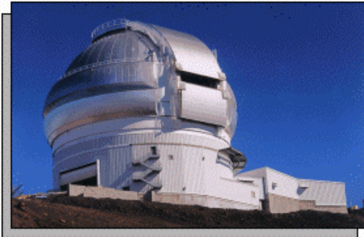
The completed Gemini North enclosure and dome.
