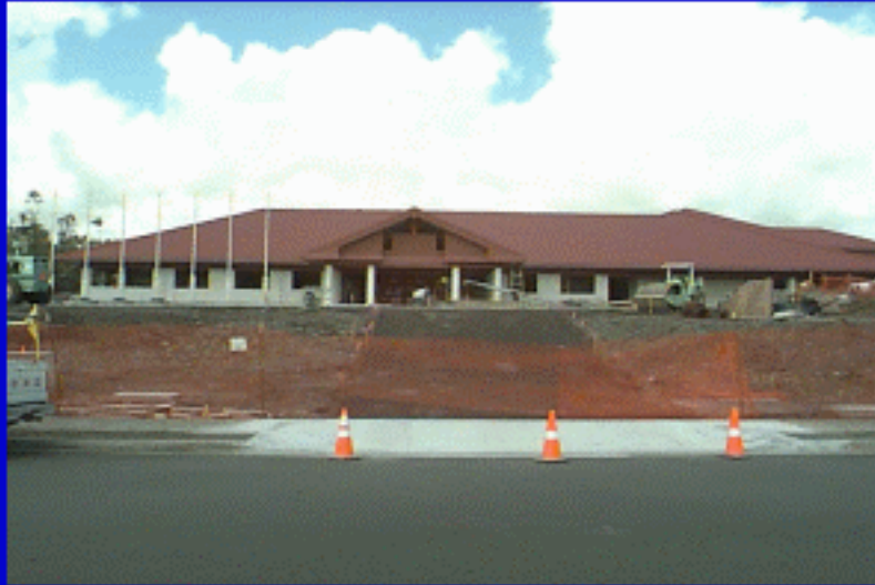
Construction of the H50 Base Facility in Hawaii
