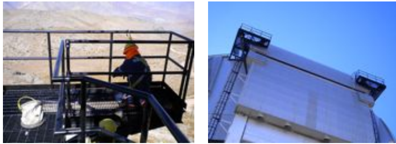
Figure 4-2: Installation of shutter drive access platforms at Gemini South.
